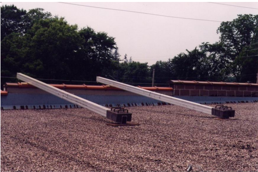
Outrigger Beam Setup
